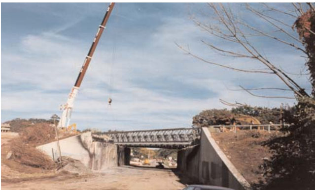
FIGURE 4 Two temporary steel panel truss bridges on I-87.
