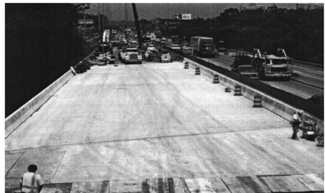
Fig. 3. Newly constructed I-95 bridge deck and detour lanes
