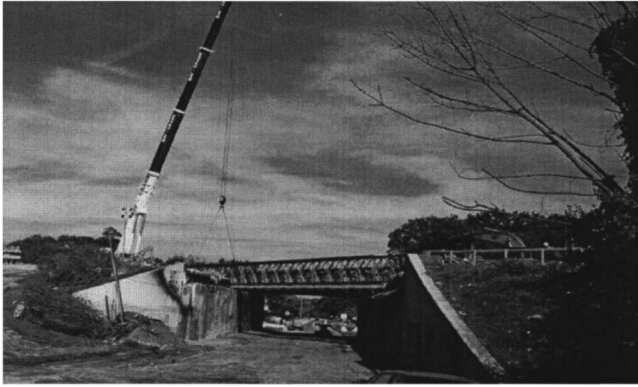
Fig. 4. Two temporary bridges on I-87
