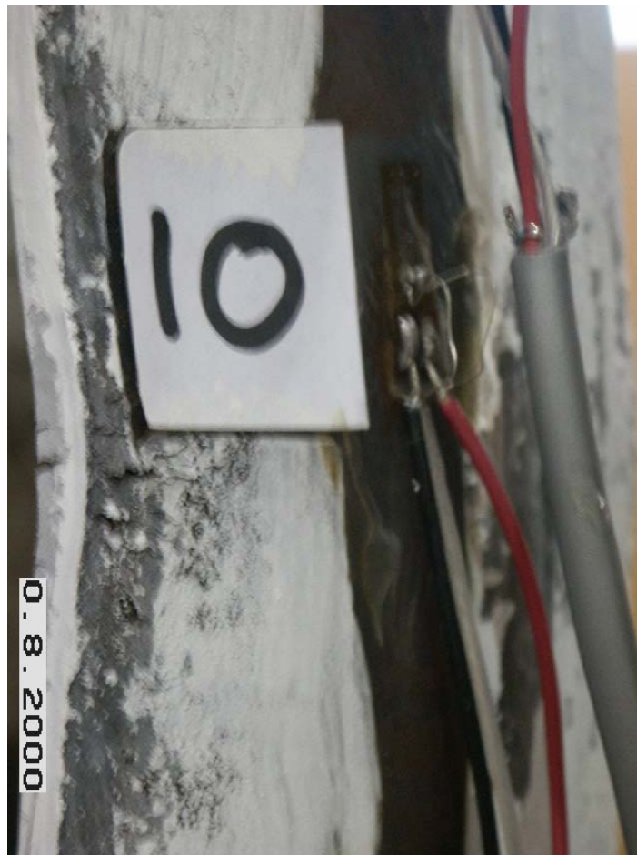
FIG. I2 – FATIGUE FAILURE CLOSE-UP FROM OUTSIDE, LOAD STEP #12, FIRST CYCLE.
