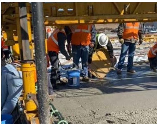
Figure 2.58: Applying Finishing Aid to the Concrete Surface
