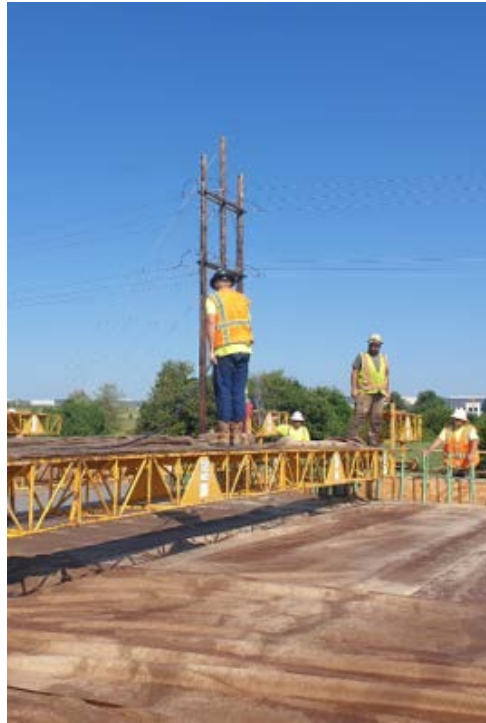
Figure 2.68: Rewetting the Burlap on the Deck
