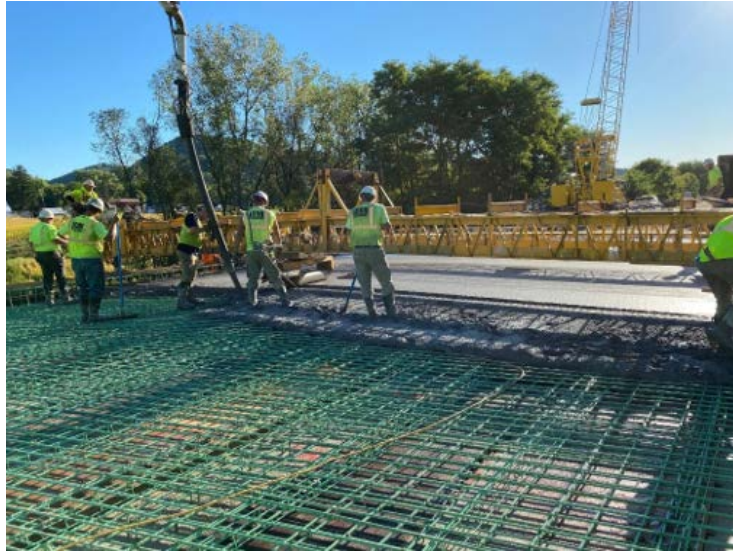
Figure 2.36: MN-IC-LC-HPC-9 Placement
