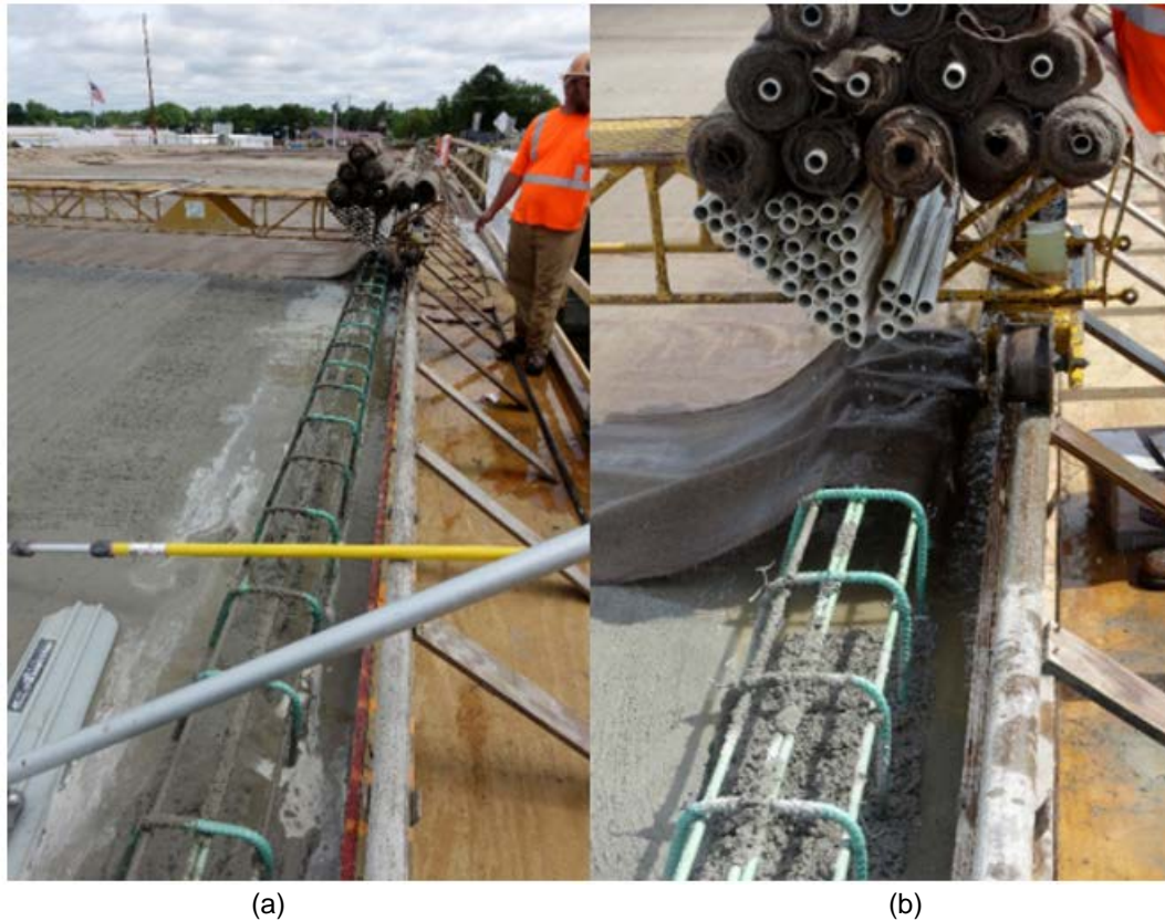
Figure 2.6: Water from Burlap Dripping onto the Deck (a) An Overview; (b) A Close-Up View
