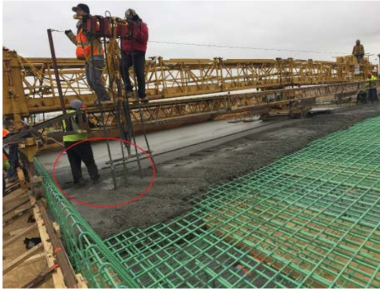
Figure 2.46: Walking Through Consolidated Concrete
