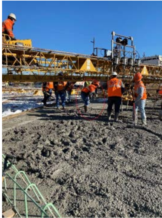
Figure 2.56: Walking Observed on Freshly Consolidated Concrete
