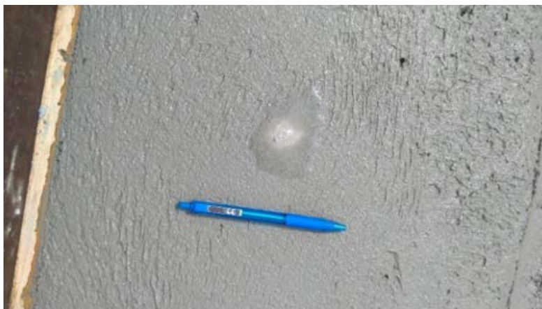
Figure 2.26: The Appearance of Air Pockets on the Concrete Surface (Image Provided by MnDOT)
