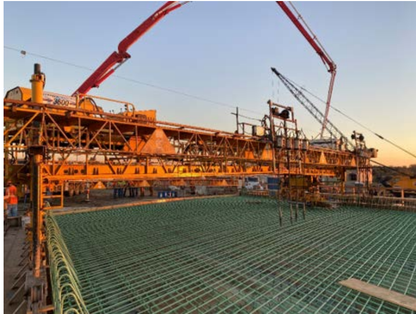
Figure 2.50: Consolidation and Finishing Equipment
