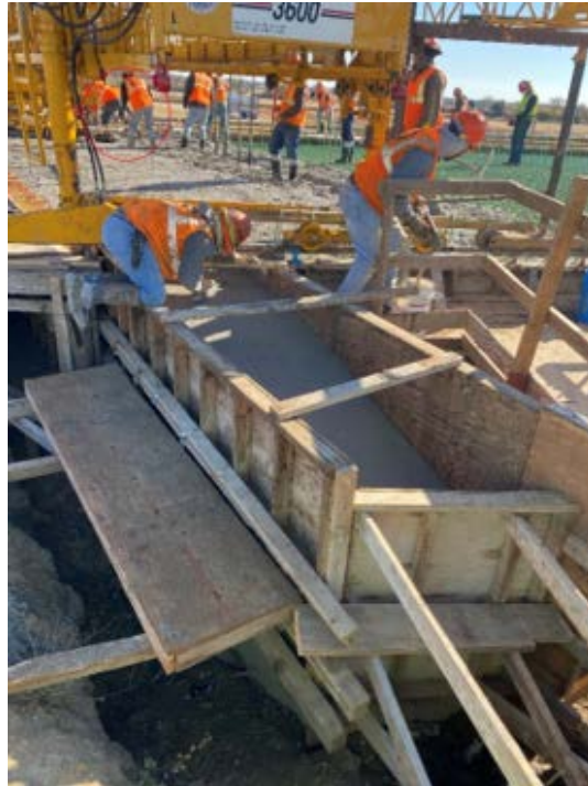
Figure 2.51: Walking Observed on Freshly Consolidated Concrete
