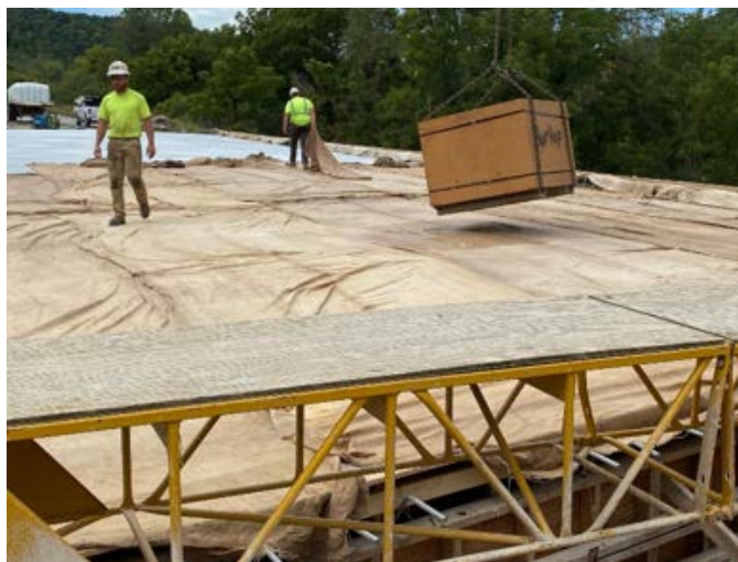
Figure 2.40: Wet Curing Application on MN-IC-LC-HPC-9
