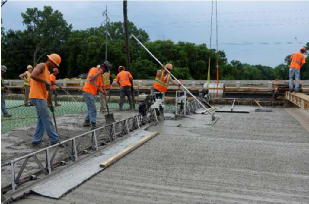
Figure 2.3: Finishing Equipment for MN-IC-LC-HPC-2 Subdeck
