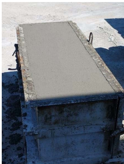
Figure 2.27: Placement of Second Truckload in Second Trial Placement (Containing Set Retarding Admixture) with No Observable Air Pockets on the Concrete Surface
