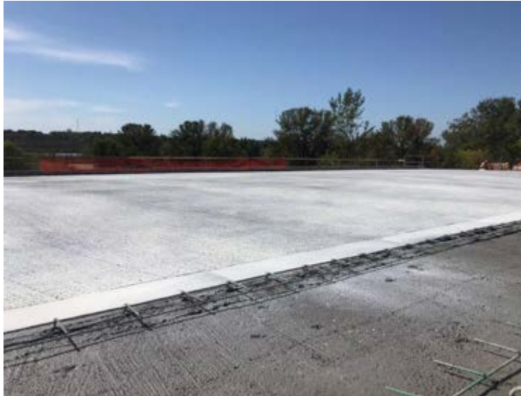
Figure 2.20: The Application of the Curing Compound on the Roadway of the Deck Showing Uneven Coverage
