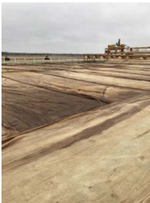
Figure 2.48: Burlap Placement on the Deck
