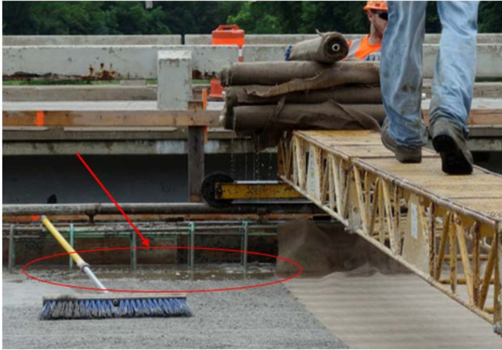
Figure 2.4: Water from Burlap Dripping onto the Deck
