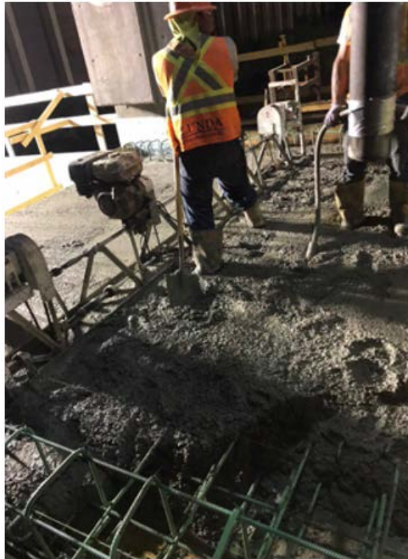
Figure 2.10: Placement, Consolidation, and Finishing of MN-IC-LC-HPC-5
