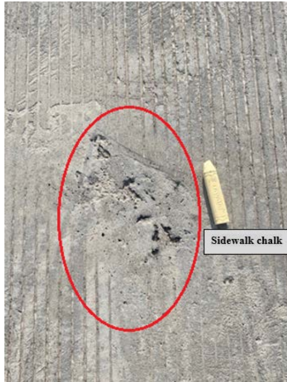
Figure 3.34: Surface Damage Observed on KS-IC-LC-HPC-2-P1
