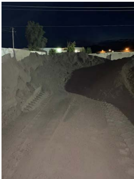
Figure 2.35: Disturbance of the Bottom of the Stockpile
