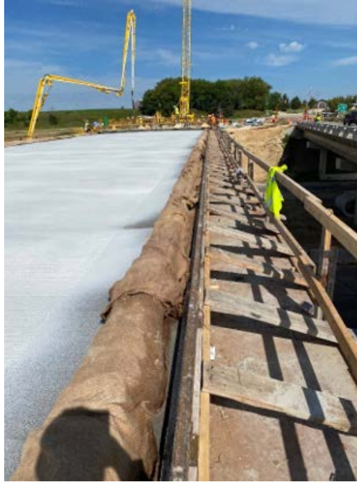
Figure 2.33: Burlap Placement on the Barrier Reinforcement
