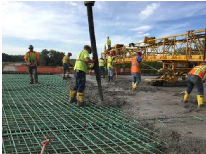
Figure 2.18: Walking Through Consolidated Concrete
