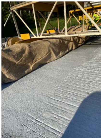
Figure 2.38: Burlap Placement on the Barrier Reinforcement
