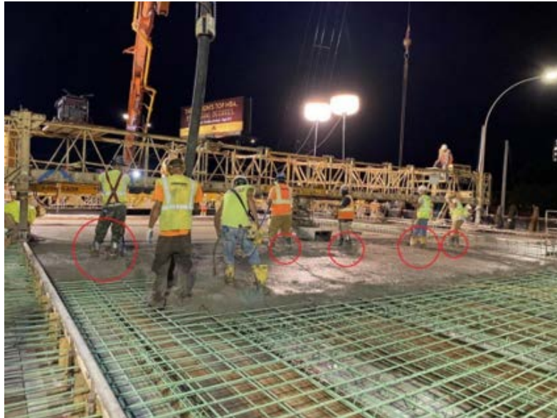
Figure 2.23: Walking Observed on Freshly Consolidated Concrete
