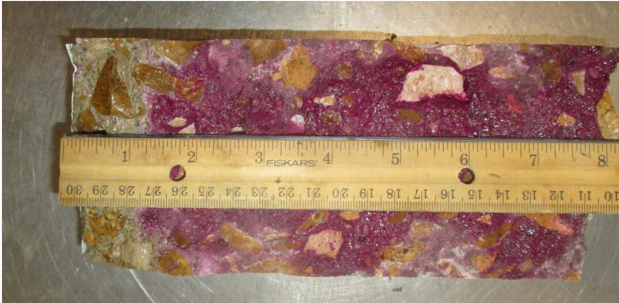
Figure 6: Carbonation depth for Core B4
