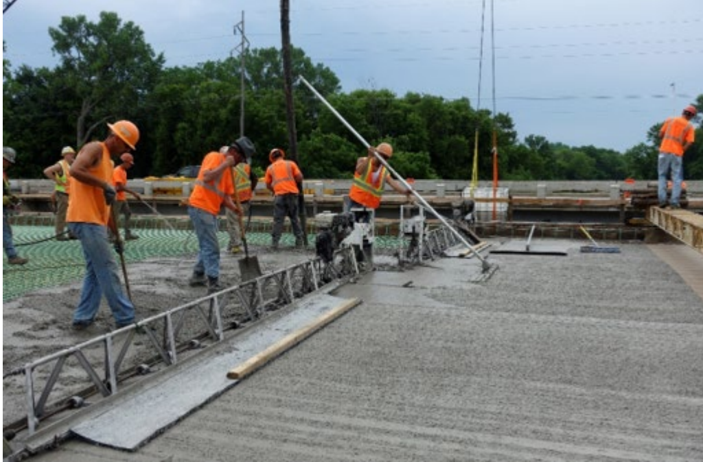
Figure 4.2: Finishing equipment for MN-IC-LC-HPC-2 subdeck
