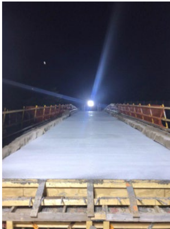
Figure 4.13: The application of the curing compound on the bridge deck
