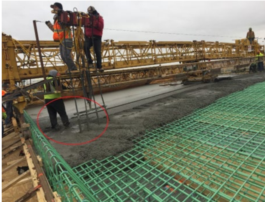
Figure 4.46: Walking through consolidated concrete
