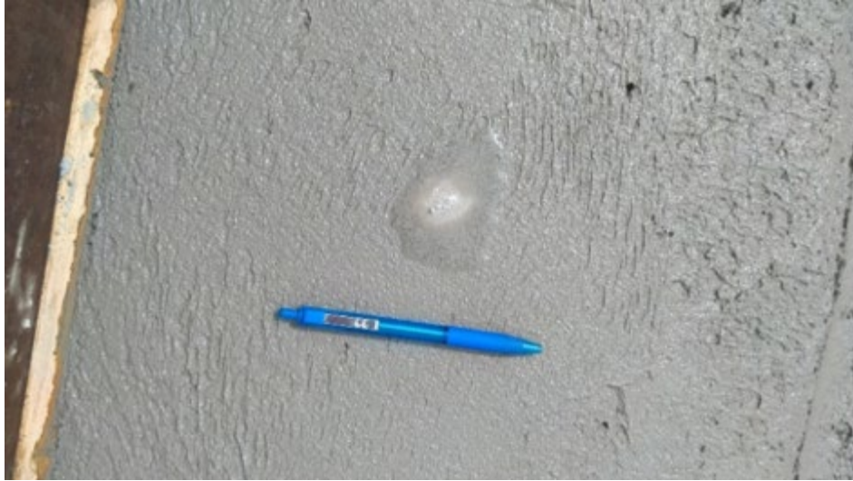
Figure 4.25: The appearance of air pockets on the concrete surface (image provided by MnDOT)
