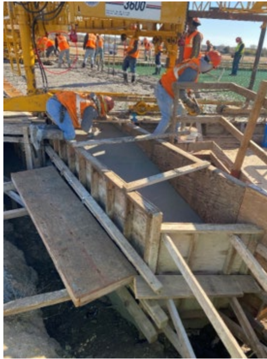
Figure 4.51: Walking observed on freshly consolidated concrete
