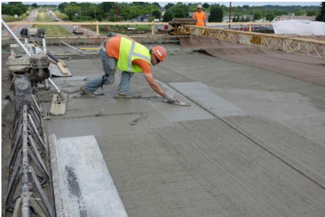
Figure 4.4: Walking through freshly consolidated concrete
