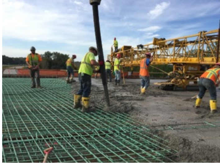
Figure 4.17: Walking through consolidated concrete
