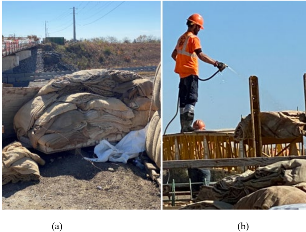
Figure 4.54: Burlap placement of KS-IC-LC-HPC-2 (a) dry burlap; (b) wetting the burlap on the deck
