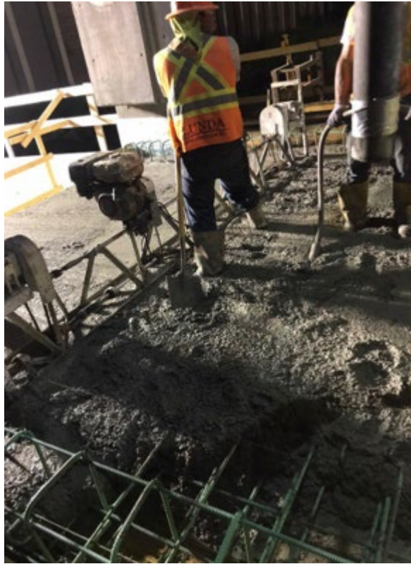
Figure 4.9: Placement, consolidation, and finishing of MN-IC-LC-HPC-5
