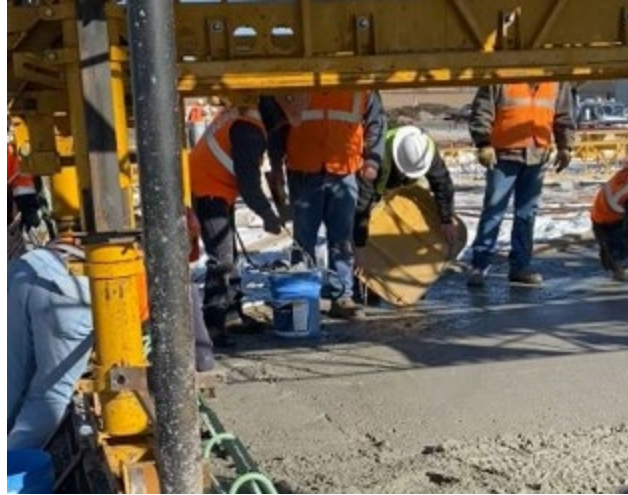
Figure 4.58: Applying finishing aid to the concrete surface
