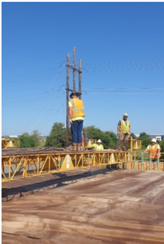
Figure 4.68: Rewetting the burlap on the deck
