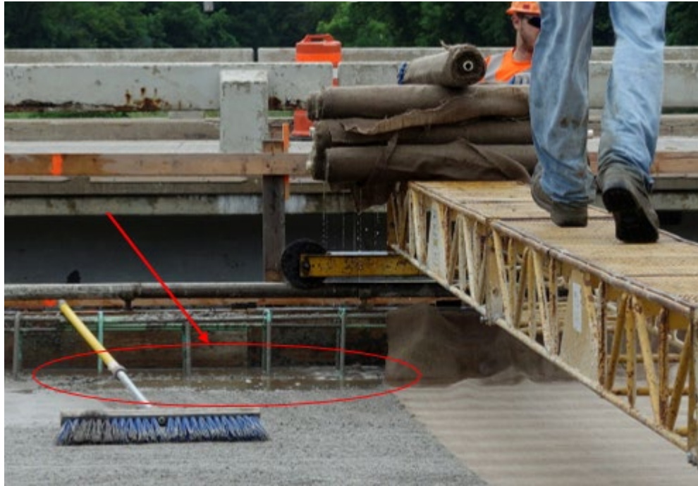
Figure 4.3: Water from burlap dripping onto the deck
