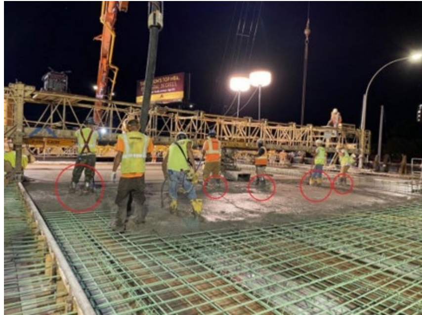
Figure 4.22: Walking observed on freshly consolidated concrete
