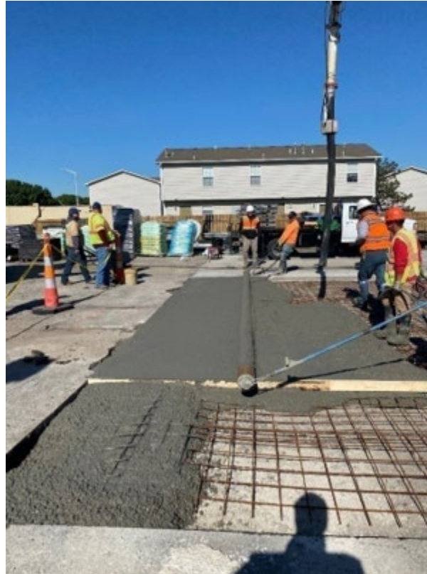
Figure 4.63: The qualification slab placement equipment
