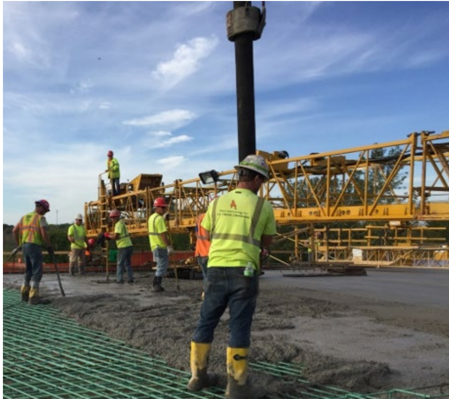
Figure 4.16: Placing, consolidation, and finishing equipment
