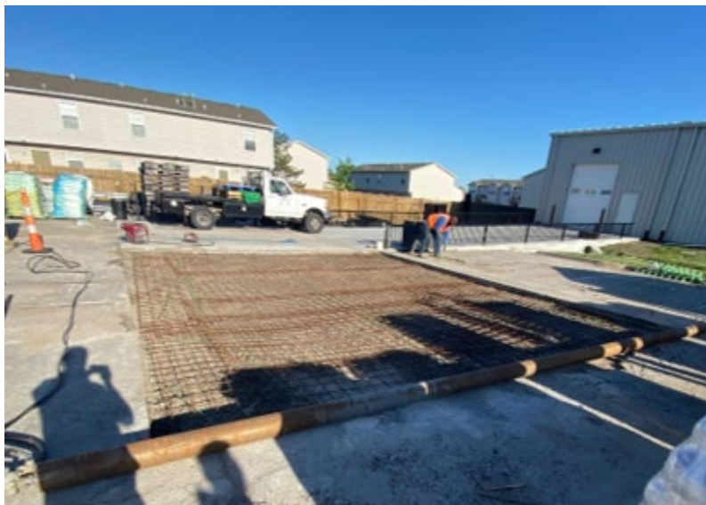
Figure 4.62: The qualification slab for KS-IC-LC-HPC-3
