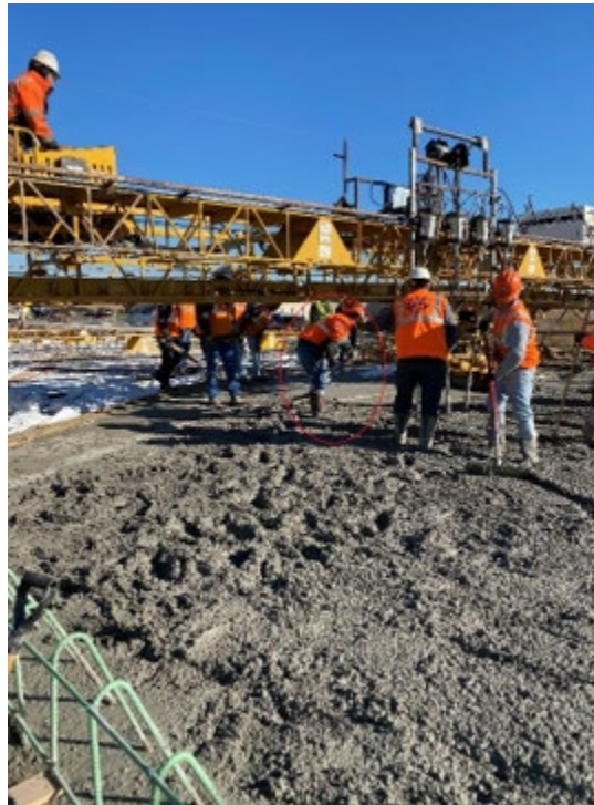
Figure 4.56: Walking observed on freshly consolidated concrete
